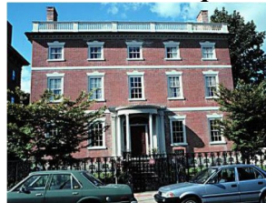
Belt Course/Projecting Cornice
